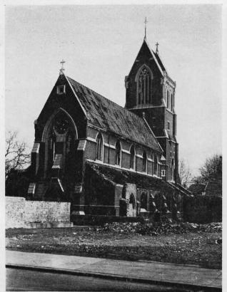
Fig. 3. St. Matthias, Stoke Newington, 1850-3. Exterior, showing the saddleback and the central buttress of the West front.
